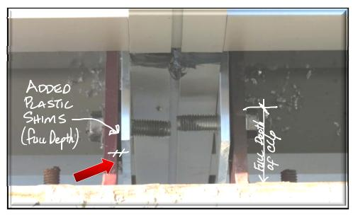
Also, it is very important that the shims they use to separate the two materials are FULL DEPTH (of clip) and SOLID around the fastener.
